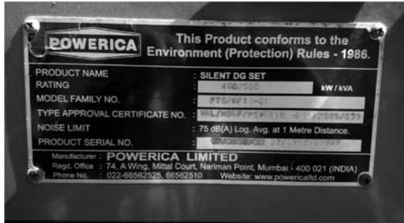
Figure 11 : Specification tag of diesel generator
