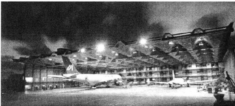
View 3: Outer View of the Hangar with One Airbus 300
