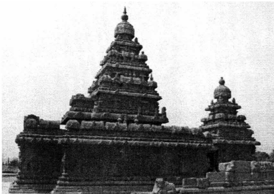
View 10: View of Temple in Dry Granite Masonry
