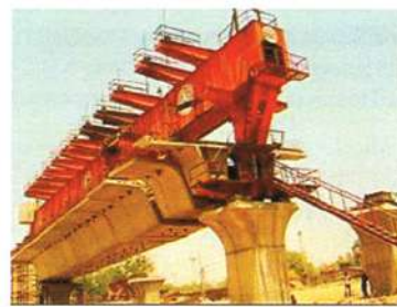
Fig 23. Erection technique for standard spans
