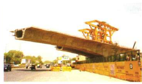
Fig 24. Simultaneous progress of both carriageways by cantilevering
