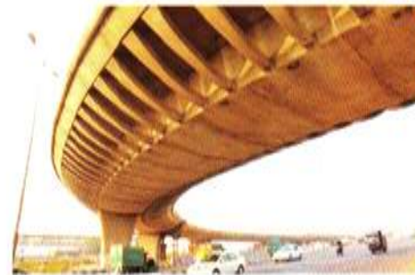
Fig 44. Spine beam with curved ribs supporting the deck cantilevers
