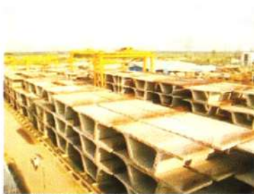
Fig 22. Barapulla stacking yard for segments
