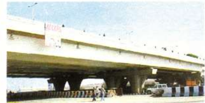
Fig 27. Mukerba chowk: continuous steel box girder with composite concrete slab
