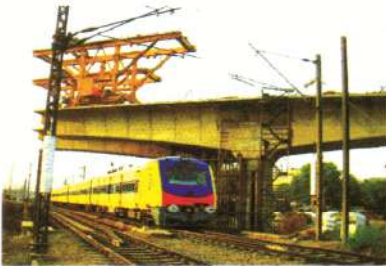
Fig 25. The Railway crossing under construction operation midnight: 2 hrs, alternate days
