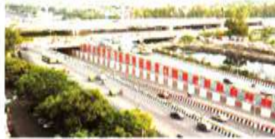
Fig 4. Completed structure: Flyover by free cantilever ; Underpass by diaphragm wall
