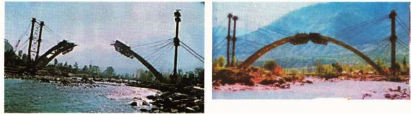
Fig 35. Parvati bridge: Arch construction by free cantilevering
