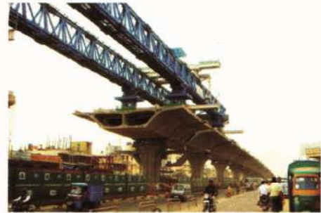
Fig 37. Bangalore Hosur expressway: Precast segmental construction erection by overhead launching truss
