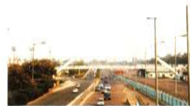
Fig 8. FOB crossing Barapulla elevated road near Jln stadium
