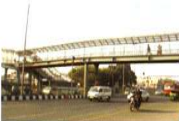
Fig 6. Typical footbridge in Delhi: Median support is vulnerable
