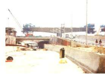
Fig 19. Free cantilevering of bridge during construction of subway
