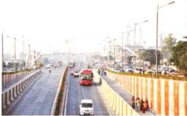
Fig 17. Ghazipur interchange showing pedestrian path-cum – cycle track and FOB
