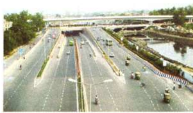
Fig 18. Ghazipur interchange showing main constituents
