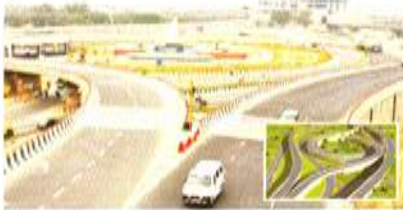
Fig 3. Badarpur elevated corridor, New Delhi • minimise structure, maximise embankments • landscaping • reduced environmental impact by depressing interchange
