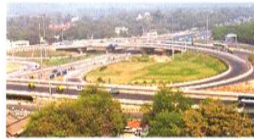
Fig 2. Innovative grade separation at Safdarjung-AIIMS, Delhi • Signal free junction • Landscaping in public spaces • Reduced structure, increased earth embankments
