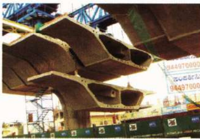
Fig 38. Precast segments suspended from main truss during erection
