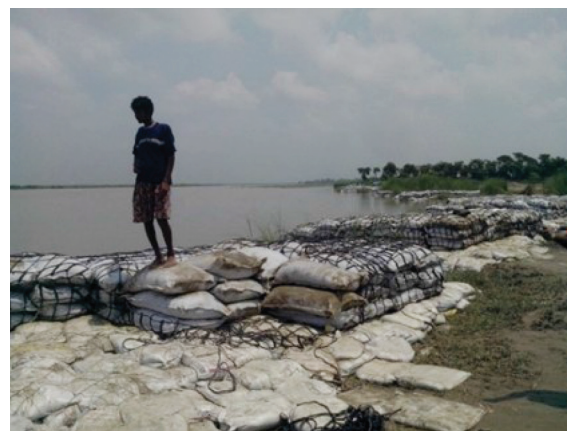
Fig. 1 Teeth Bar along the Gandak River, PD ring bandh (West Champaran, Bihar)
