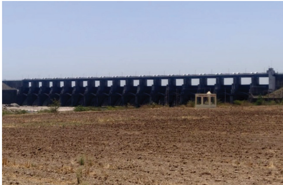
Fig. 1 Photo of Aji-III dam
