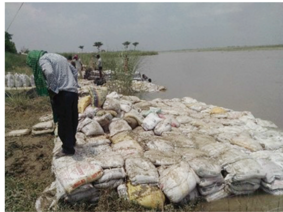
Fig. 3 Nylon crate work along Gandak river (West Champaran, Bihar)
