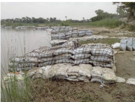
Fig. 2 Polymer rope Gabion, PD ring bandh (West Champaran, Bihar)
