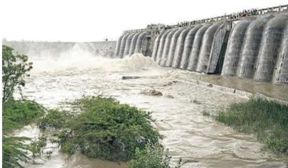
Fig. 5 Syphon Spillway of Sarala Sagar Project in Telangana
