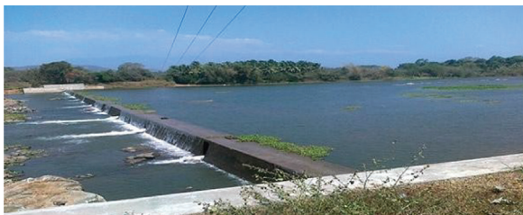
Fig. 2 Anicut across a stream overflowing the excess flood water
