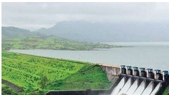
Fig. 3 Reservoir with a Spillway with gates
