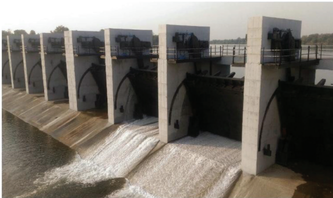
Fig. 4 Automatic falling gates in an Anicut
