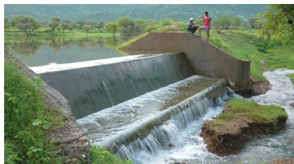
Fig. 1 Surplus Weir of a Tank overflowing the excess flood
