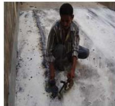
Photo 13: Thermosealing of the joints
