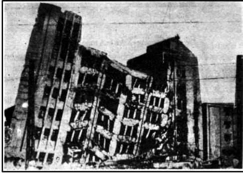
Fig 9 Failure of a Departmental store during 1948 Fukull earthquake
