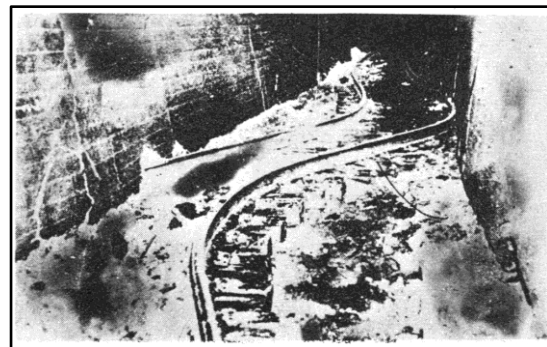
Fig 16 Large deformations of a railway track inside a tunnel
