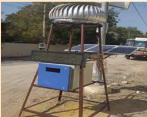
Hybrid PV and Aluminium bladed vertical axis wind turbine
