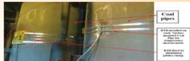
RTD mounted on coal pipe for temperature measurement
