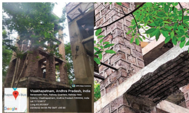
Fig 8 Cracks in stone masonry
