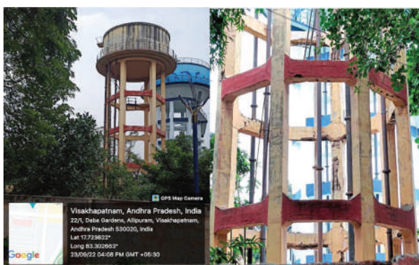
Fig 11 Damaged supports of municipal tank
