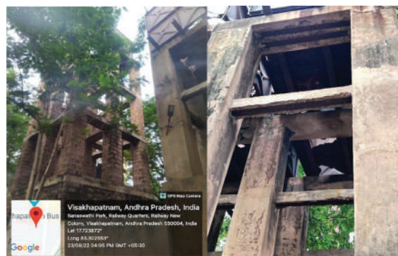
Fig 1 Practical example of deterioration of iron tank
