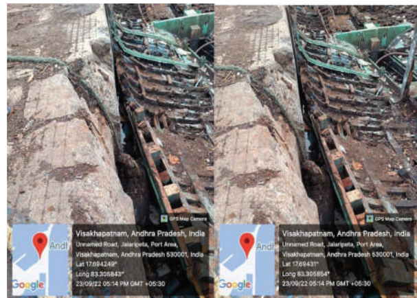
Fig 4 Wearing out of concrete
