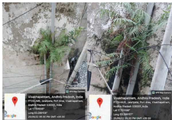
Fig 3 Growth of plant from pipe
