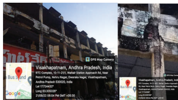
Fig 6 Spalling of column
