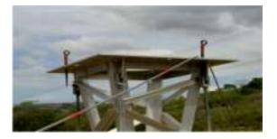
**Figure 3.6.3-7** Place box wrench in bolt holes on top of Gimbal Joint. This will keep the grip hoist cable from sliding on the Gimbal Joint during erection. Attach Grip Hoist to temporary anchor approximately 15 meters away from foundation on the opposite side from the gin pole.
