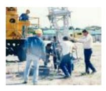
**Figure 3.6.1-4 (C)** Once the ERS Column is over the Foundation the Tie Rods on the Gimbal are released so that the bottom portion of the Gimbal can rotate. The ERS Column is lowered and the bottom flange of the Gimbal is bolted to the Foundation.
