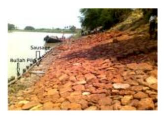
Figure 6 Sausage used to protect embankment
