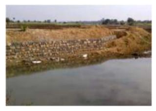
Figure 8 Gabion wall used to protect embankment
