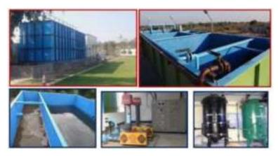
Figure 5 New 100 KLD STP with MBBR Technology
