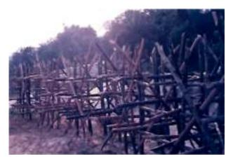
Figure 3 Bamboo porcupines (making in progress)
