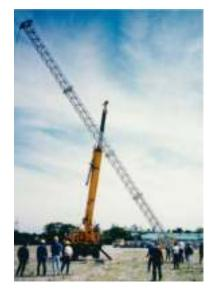
**Figure 3.6.1-4 (B)** The ERS Column and Gimbal is walked in toward the Foundation.
