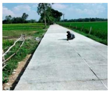
Figure 2 Good quality village concrete road in Amethi district prepared with conventional curing technique for 7 days
