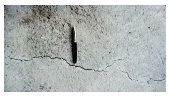
Figure 1 A typical plastic shrinkage crack [6]
