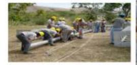
(B) Slide together over connection splice
