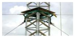
**Figure 3.6.3-20** The slings must go around one or more of the  $3'' \times 3''(76 \text{ mm} \times 76 \text{ mm})$  main vertical angles.
