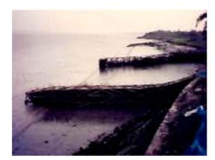
Figure 4 Semi permeable spur
