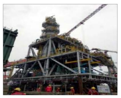
Figure 5 Module with conventional deaeration tower
