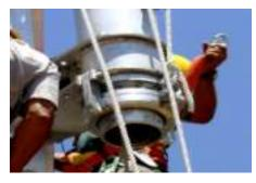
**Figure 3.6.3-17** Once the mast has been raised to the top, place the two keeper bolts (or ERS Bolts) through the holes provided at the bottom of the gin pole and secure with nuts.
