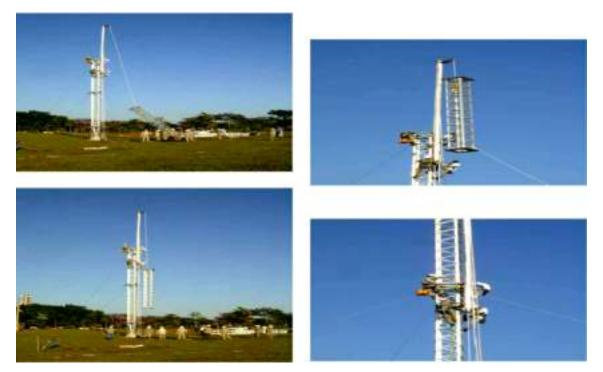
Figure 3.6.3-19 Sequence of erecting a column section.
