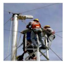
**Figure 3.6.3-11** Note the positioning ropes on the gin pole, four places used to keep gin pole centered when lifting.
