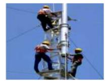
Figure 3.6.3-16 Lift the Gin Pole Mast
