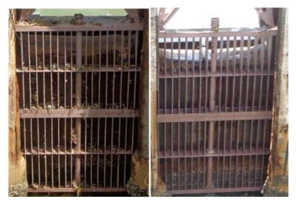
Figures 2 AFC applied screen (a) before cleaning (b) after cleaning
