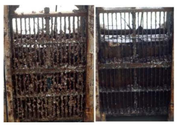
Figures 3 Non-AFC screen (a) before cleaning (b) after cleaning
