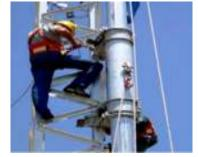
**Figure 3.6.3-14** Turn the slider and close the swing clamps around the large angle.
