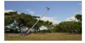
**Figure 3.6.3-8** Tension grip hoist and pull gin pole in place. Note Position of davit arm. Always place vertical Note the Positioning Ropes, 4 Places used to keep gin pole centered when lifting
