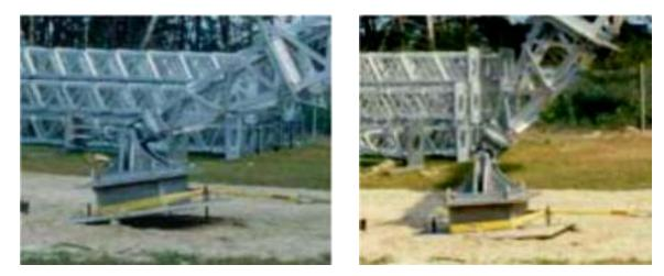
**Figure 3.6.2-1** When whipping up a column, or erecting a column using a gin pole, the foundation will begin to tip, since the hinge point of the gimbal is above ground level. This tipping does not present a problem and the foundation will settle down after additional vertical column weight is on the structure. The ERS computer programs will calculate the horizontal and vertical loads on the foundation
