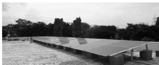
Figure 2 PV panel mounting arrangement
