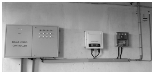
Figure 3 Solar hybrid controller, online inverter and net meter –set up
