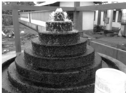
Figure 2 Cascade aerator embedded with pebbles
