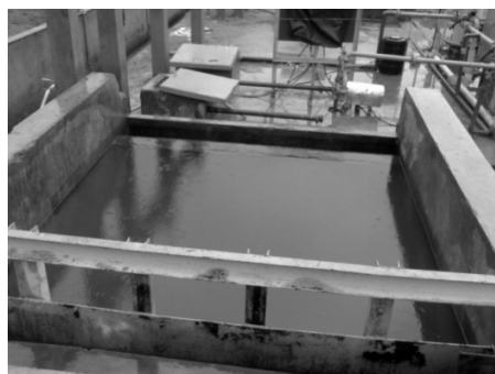
Figure 4 Gravity settling tank
