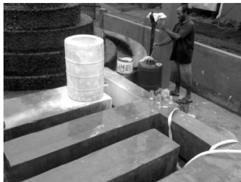
Figure 3 Mixing channel alum and lime dosing
