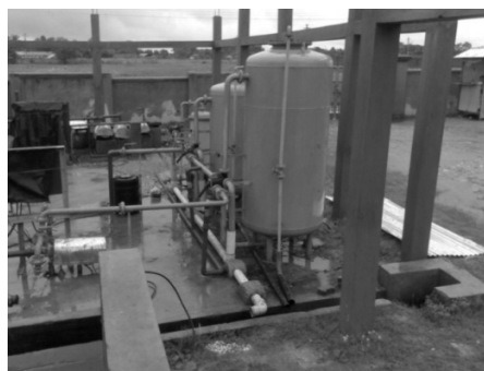
Figure 5 Catalytic iron removal filter and pressure sand filter
