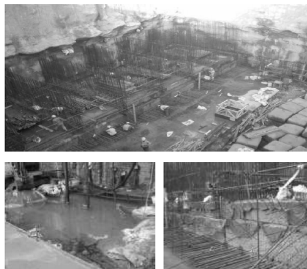
Counter Balancing of Soil Pressure, Ground water collection and Construction Joint of Bottom Raft
