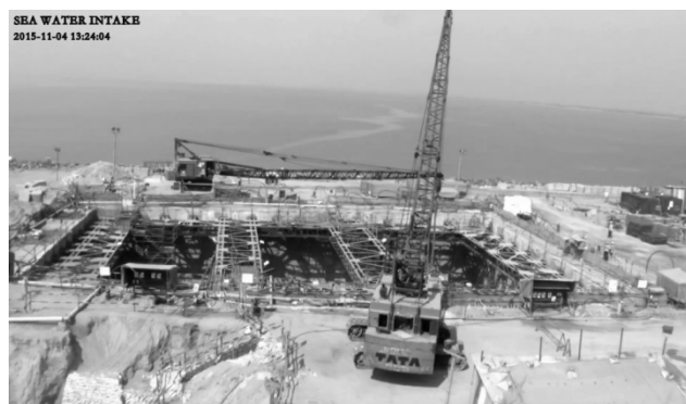
Counter Balancing of Soil Pressure, Ground water collection and Construction Joint of Bottom Raft
