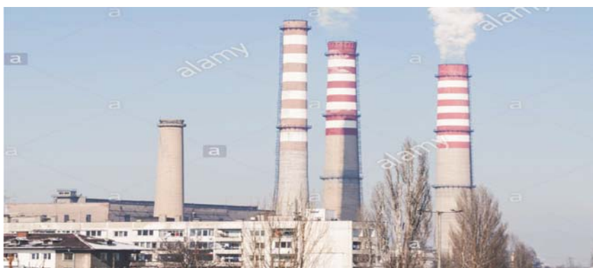
Photo of the Thermal Power Station
