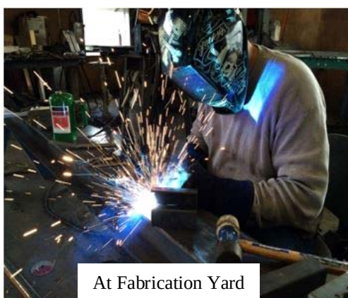
Fig. 1 Examples of some on-site welding
